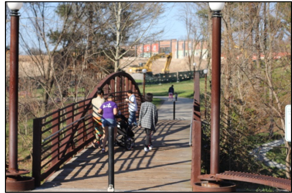
Pedestrian Bridge (AECOM, 2015)
