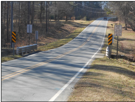
Sedalia Road (Bridge #400207) (AECOM, 2015)
