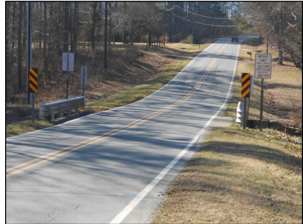
Existing conditions on Sedalia Road (AECOM, 2015)
